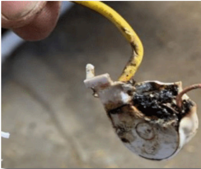
Damaged light connector.
